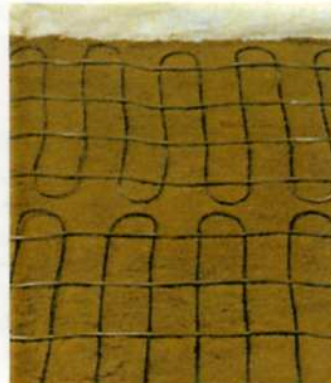
Fixtherm-Heizmatte FS 10 ausrollen ...
