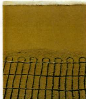
... Fixtherm-Heizmatte FS 5 ausrollen ...
